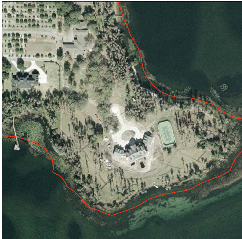
Figure 11. 2005 color Aerial shows peninsula above after construction of a private home and removal of Cypress fringe.
